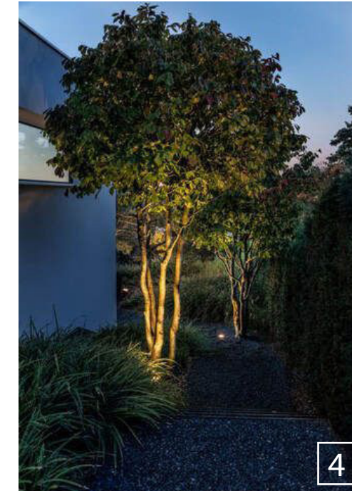
TREE UPLIGHTING STAKE MOUNTED ADJUSTABLE ACCENTLIGHTS TO UP- LIGHT THE UNDERSIDE OF TREE CANOPY
